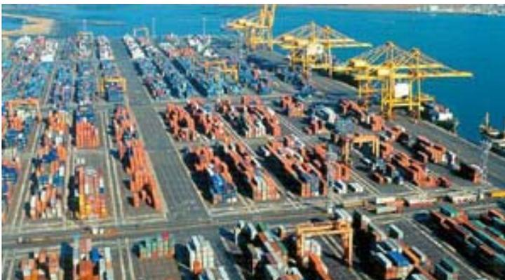
**Figure 1.** A land-scarce container terminal: stackyard, TTs (foreground), QCs (upper right).
